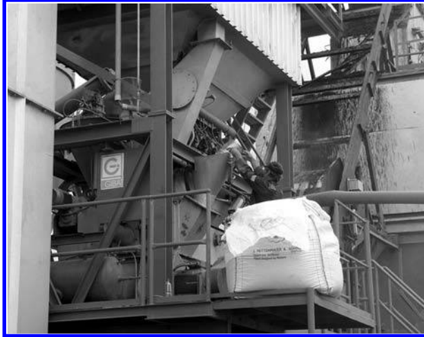
FIGURE 9.8 Manual proportioning control of a granulated stabilizer directly into the pugmill. (Photo courtesy of Bartosz Wojczakowski.)
