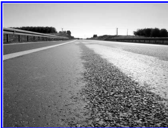
FIGURE 11.2 SMA mixture segregation—separation of mastic from coarse aggregates. (Photo courtesy of Krzysztof Błażejowski.)
