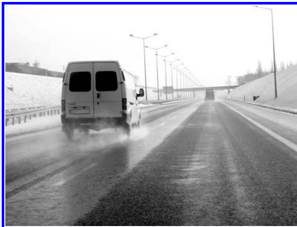
FIGURE 12.7 Water mist picked up by vehicles driving along a wet SMA pavement is reduced. (Photo courtesy of Krzysztof Błażejowski.)
