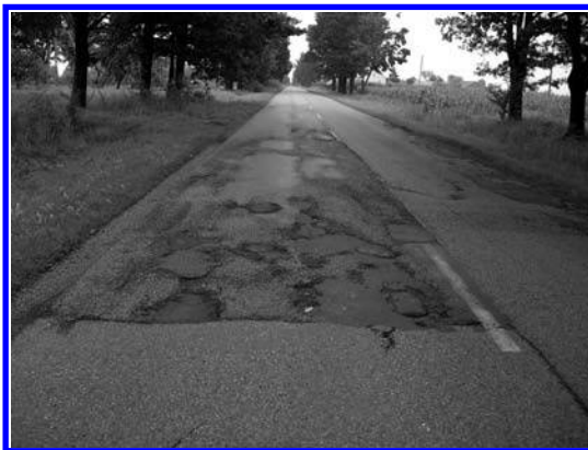
FIGURE 11.25 Beginning of a work site—effect shown years later, a consequence of spreading too cool a mixture at the beginning of the work site. (Photo courtesy of Krzysztof Błażejowski.)
