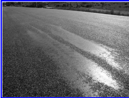
FIGURE 11.1 Longitudinal fat spots of binder. (Photo courtesy of Bartosz Wojczakowski.)
