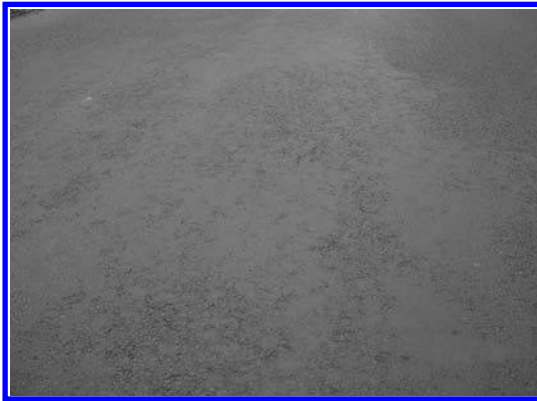
FIGURE 11.8 The closed structure of an SMA course over a large area. (Photo courtesy of Krzysztof Błażejowski.)
