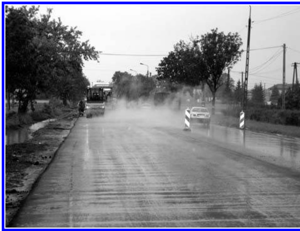
FIGURE 10.4 Laying down SMA during rainfall is not a desirable (and is mostly a forbidden) practice. (Photo courtesy of Krzysztof Błażejowski.)
