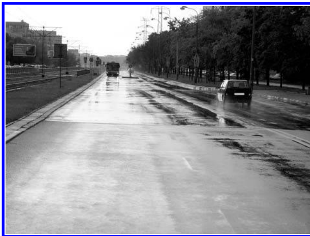
FIGURE 12.9 Differences in pavement abilities to discharge water—the SMA course ( near ) and the old dense asphalt concrete ( far ). The light reflection off the wet SMA course is substantially less than that off the asphalt concrete course. (Photo courtesy of Krzysztof Błażejowski.)
