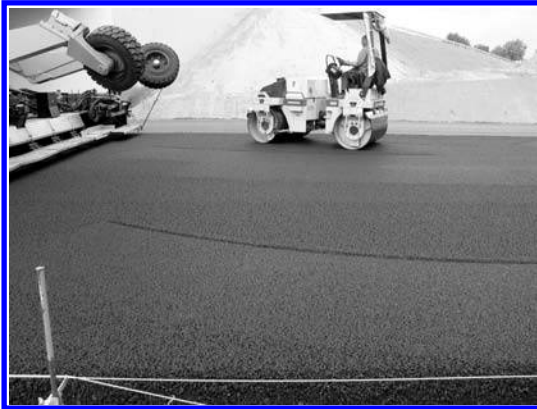
FIGURE 10.11 The particular way rollers approach the paver, with a turn being made right behind the paver. (Photo courtesy of Konrad Jabłoński.)
