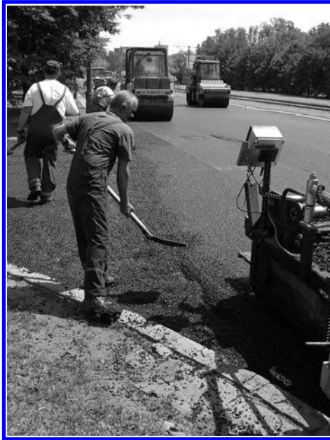
FIGURE 11.26 Manual spreading of the SMA mixture on a down ramp from a side street. (Photo courtesy of Krzysztof Błażejowski.)
