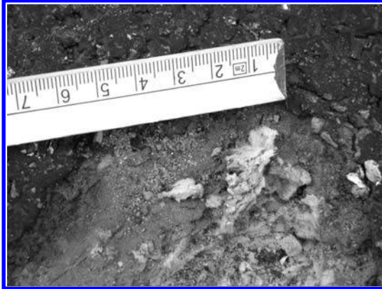
FIGURE 11.7 Stabilizer lumps incorporated into an SMA course. (Photo courtesy of Marco Schünemann.)
