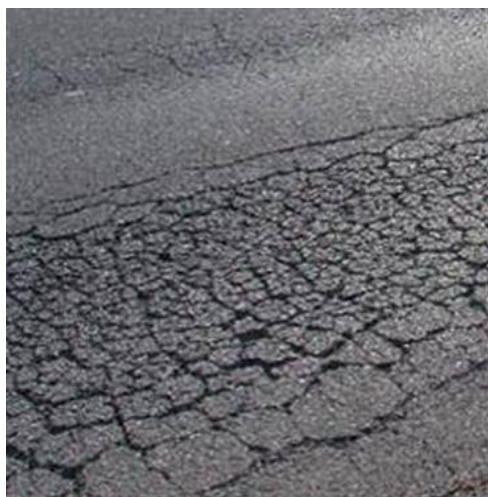
Fatigue Cracking
